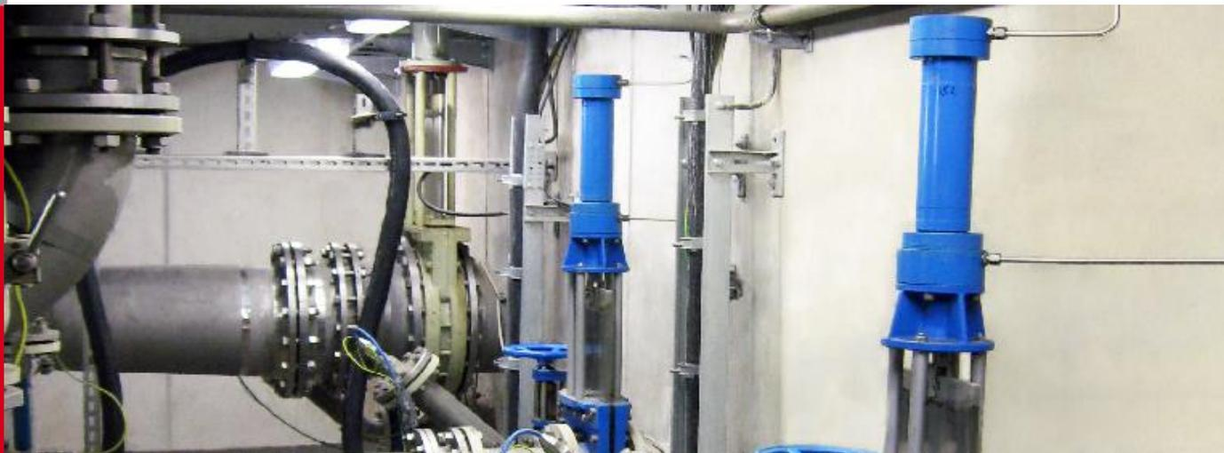
In many hydraulic applications the user needs reliable information about whether a hydraulic cylinder has reached one of its end positions. Usually this is achieved through different types of position switches (inductive, roller and switch, etc.).
